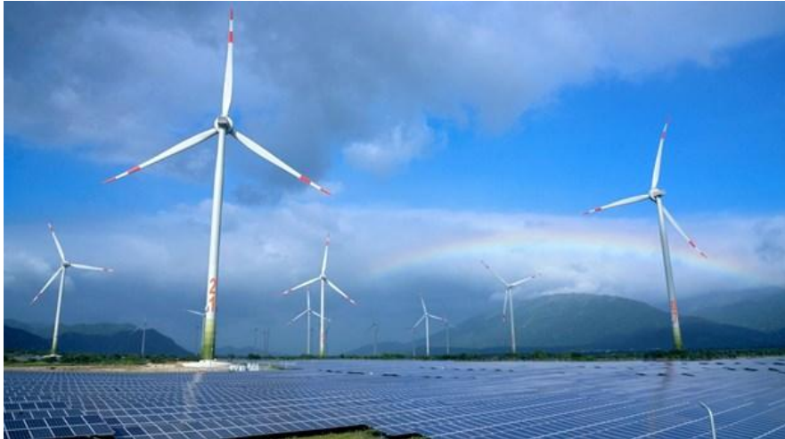
The wind and solar power plant project in Loi Hai and Bac Phong communes of Thuan Bac district has been carried out quickly thanks to support from Ninh Thuan province's authorities
