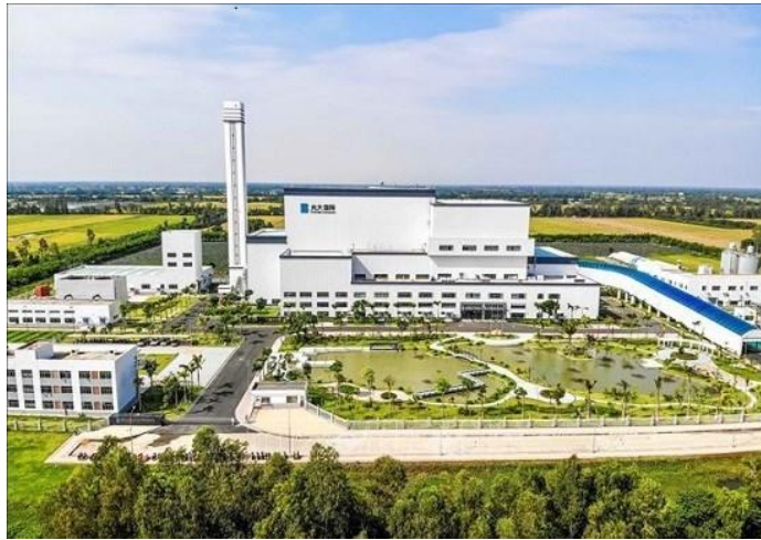
At the Can Tho waste-to-power plant in Thoi Lai district
