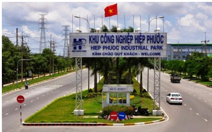
Hiệp Phước Industrial Park in Nhà Bè District. Industrial parks and processing zones in HCM City are attracting more and more investments despite COVID-19
